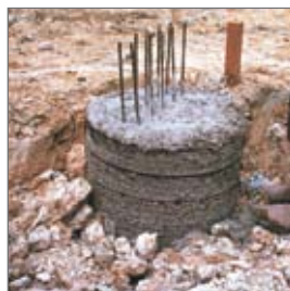
Coffrage cylindrique Cylindrical formwork
